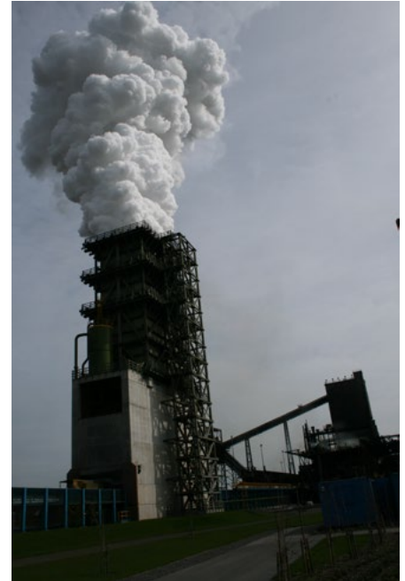
The extinguishing tower. The extreme formation of steam for about one minute is symbolic and is repeated every 10 to 20 minutes.
