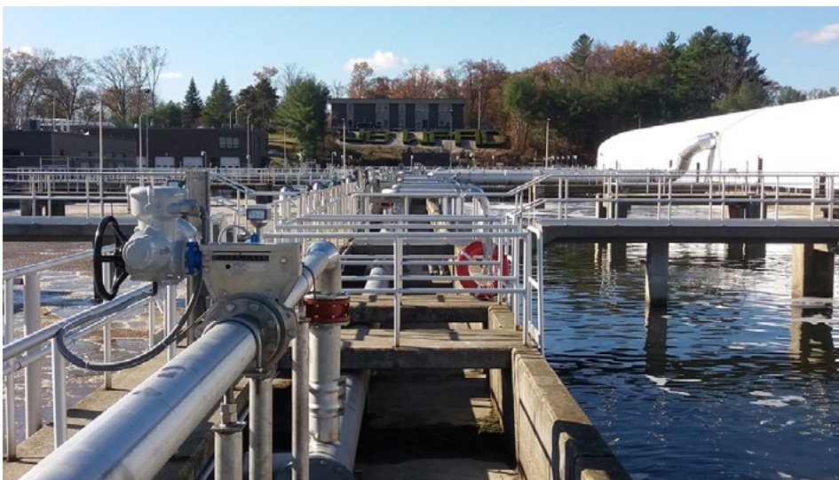
Fig. 8: Iris® diaphragm control valve with mass flow measurement at the Upper Blackstone wastewater treatment plant
